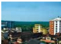
Hospital complex at Kottakkal
