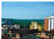
Hospital complex at Kottakkal
