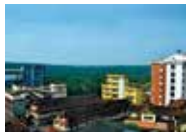
Hospital complex at Kottakkal
